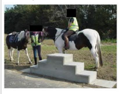
Shows the roadside mounting blocks (which had to be provided to enable horses to be lead across the bridge after a miscommunication in the design – it should have been designed to DMRB standards to allow horses to be ridden across this bridge).
