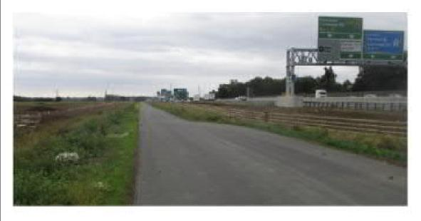
A new single track "road2 giving the home/landowners alongside north side of A14 access to and from their property. It has a wide soft vegetative verges both sides and the tarmac is as above. It is well set back from and fenced from both the A1307 and A14 (to right in this photo).
